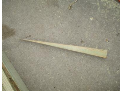
Figure A8. Cut 3 wedges for TA stringers.
