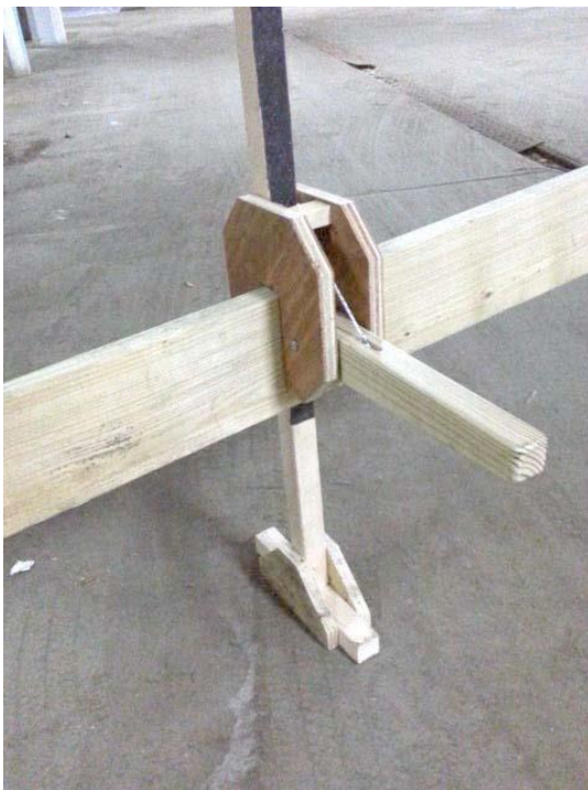
Figure E2. Frame and stringer support jigs. These are 2 types of jigs that hold the 2x6 frame or stringer while the ramp is being aligned and the posts are installed.
