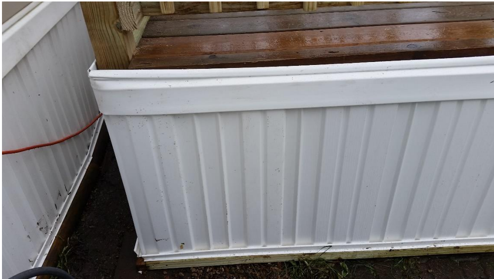
Figure D6. Completed skirting.
