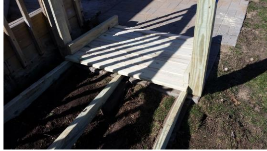
Figure 7. Stringers into Ramp end post assembly.
