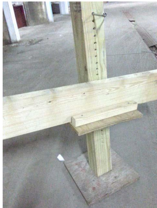
Figure E2. Frame and stringer support jigs. These are 2 types of jigs that hold the 2x6 frame or stringer while the ramp is being aligned and the posts are installed.
