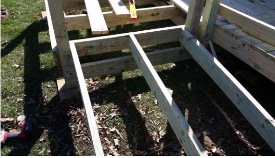
Figure 6. Ramp frame with 180° landing. Notice cross bracing
