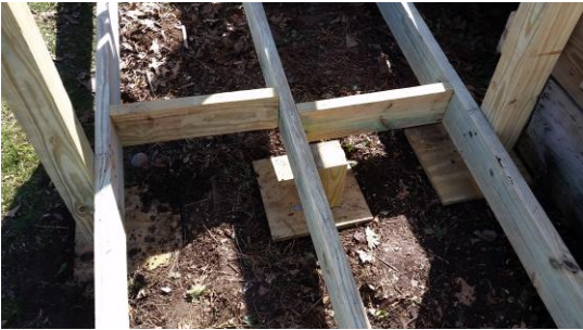
Figure 8. Ramp frame. Notice cross braces.
